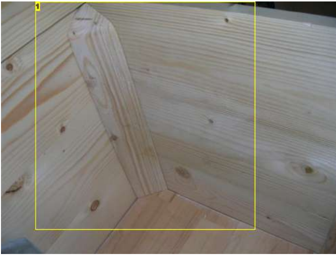
Image Notes 1. Corner support angle glued in place
