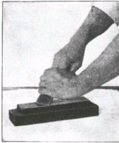
Fig. 196.—Sharpening Plane Iron.
