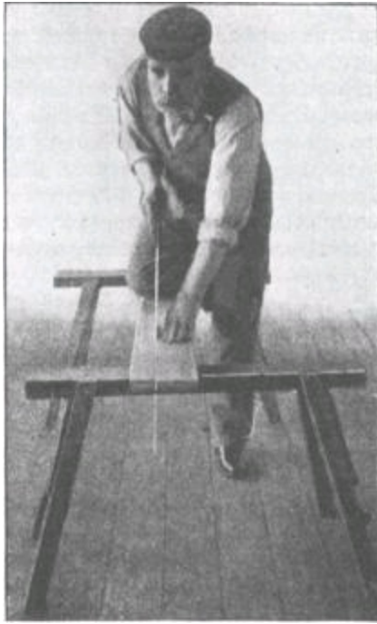
Fig. 316.—Ripping Plank, End View.
