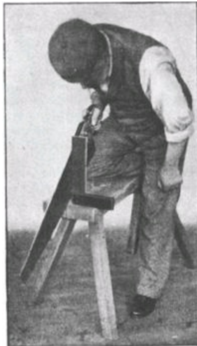
Fig. 313.—Testing Saw with Square.
