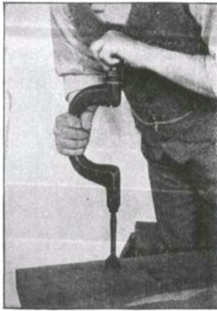
Fig. 401.—Vertical Boring with Brace.
