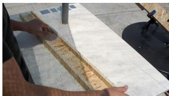
Step 19: After the piece of the fence has dried, it's time to cut the extra piece of plywood.
